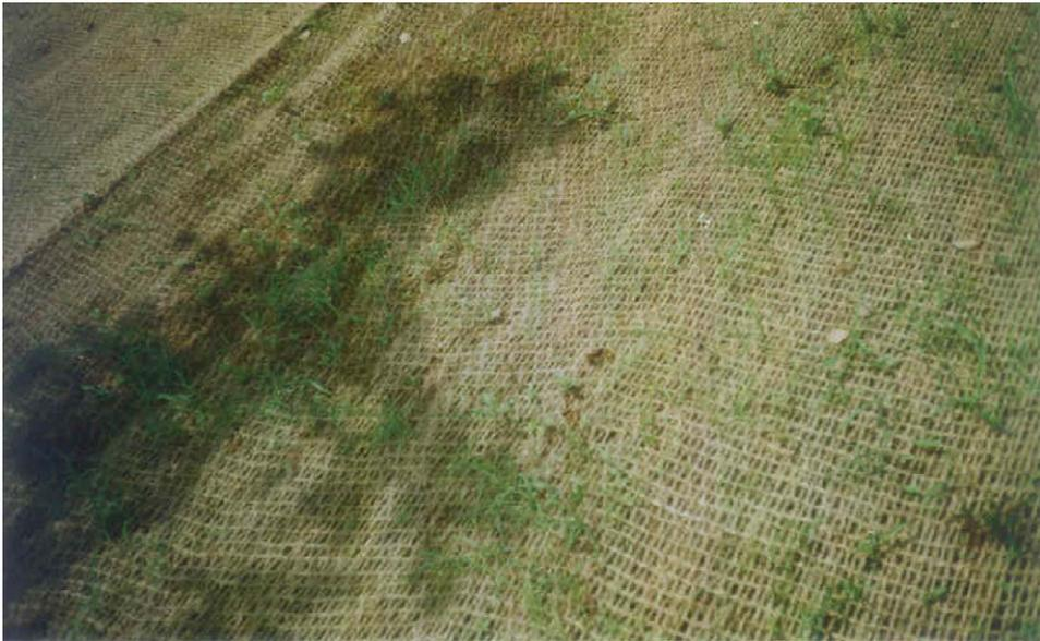
Plate 2. View of the coir geotextile laid vegetated slope after one month.
