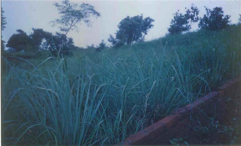
Plate 3. View of the coir geotextile laid vegetated slope after one year.
