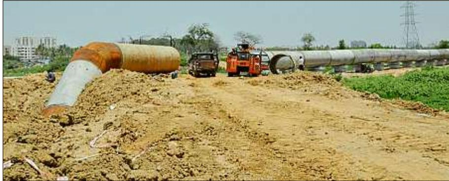
**A mud road being laid through the Varthur Lake for laying a pipeline.** DH FILE PHOTO
