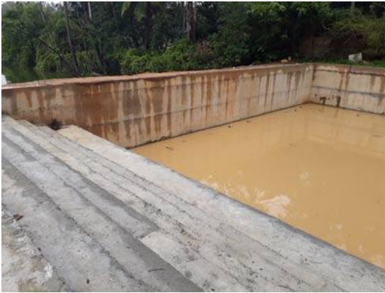
The walls in the new pond in the tank
